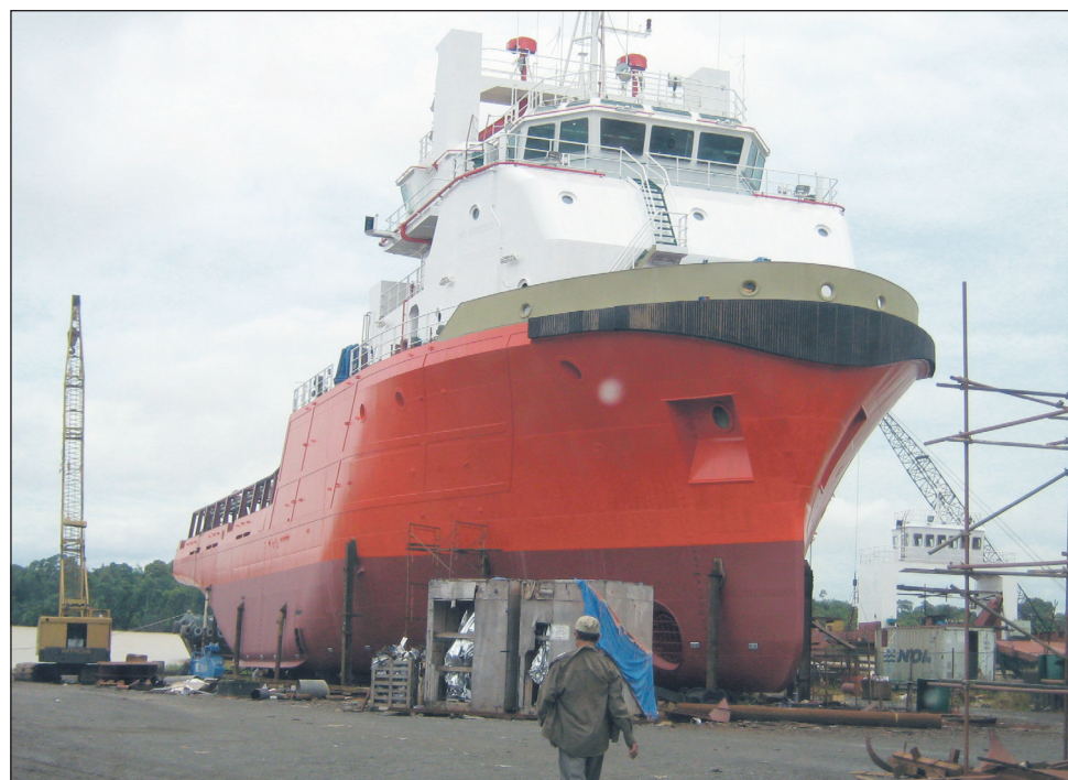
A 42-metre AHT under construction in a Southeast Asian shipyard
